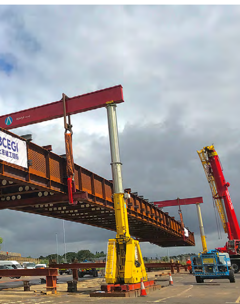
Pre-assembled offsite, a 78.5m-long section of the bridge was installed in one piece
