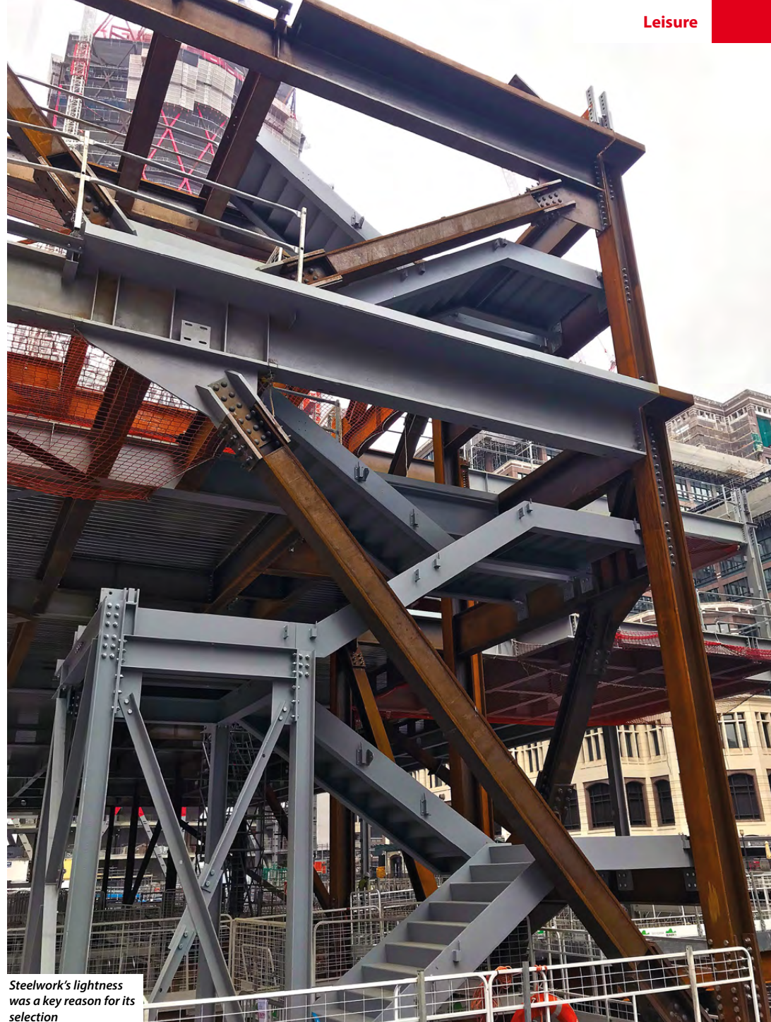
The structure sits over a dock and reuses existing piles
