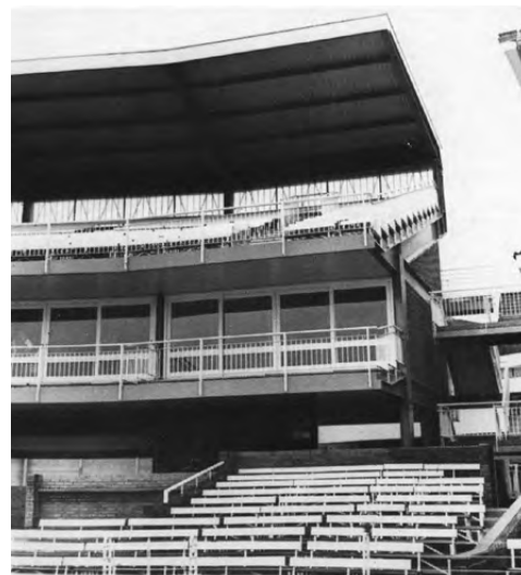
A close-up view of the new stand showing the interesting roof structure, also the terraced decking in course of construction. The use of 5/16 in thick steel plate for the decking is an unusual feature.
