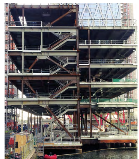
Bracing arrangement
