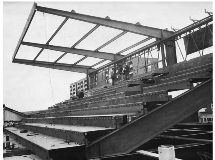
A close-up view of the new stand showing the interesting roof structure, also the terraced decking in course of construction. The use of 5/16 in thick steel plate for the decking is an unusual feature.
