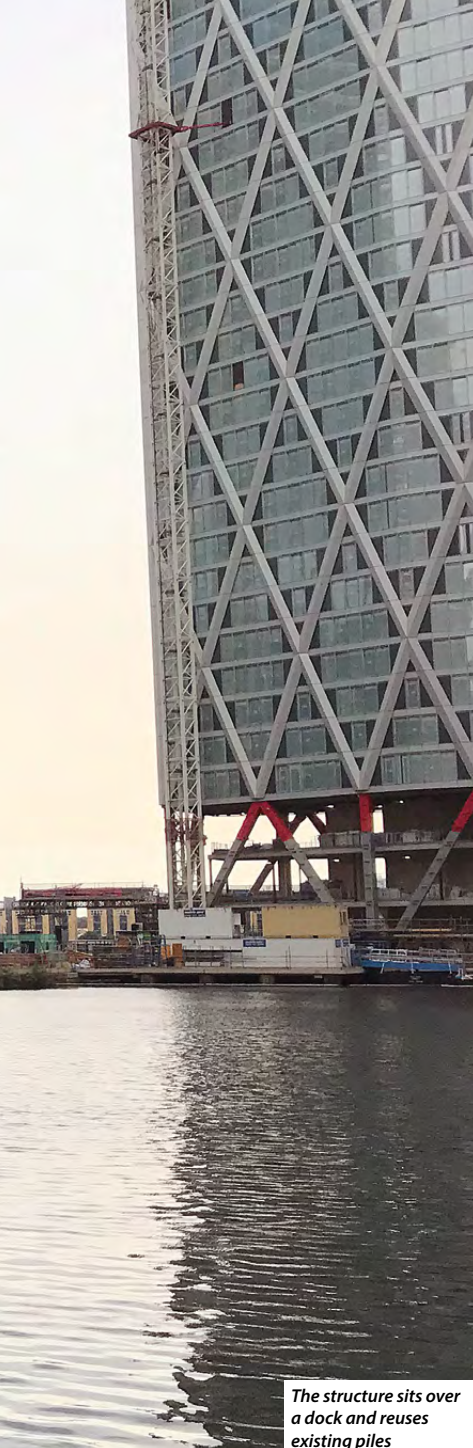
Steelwork's lightness was a key reason for its selection
