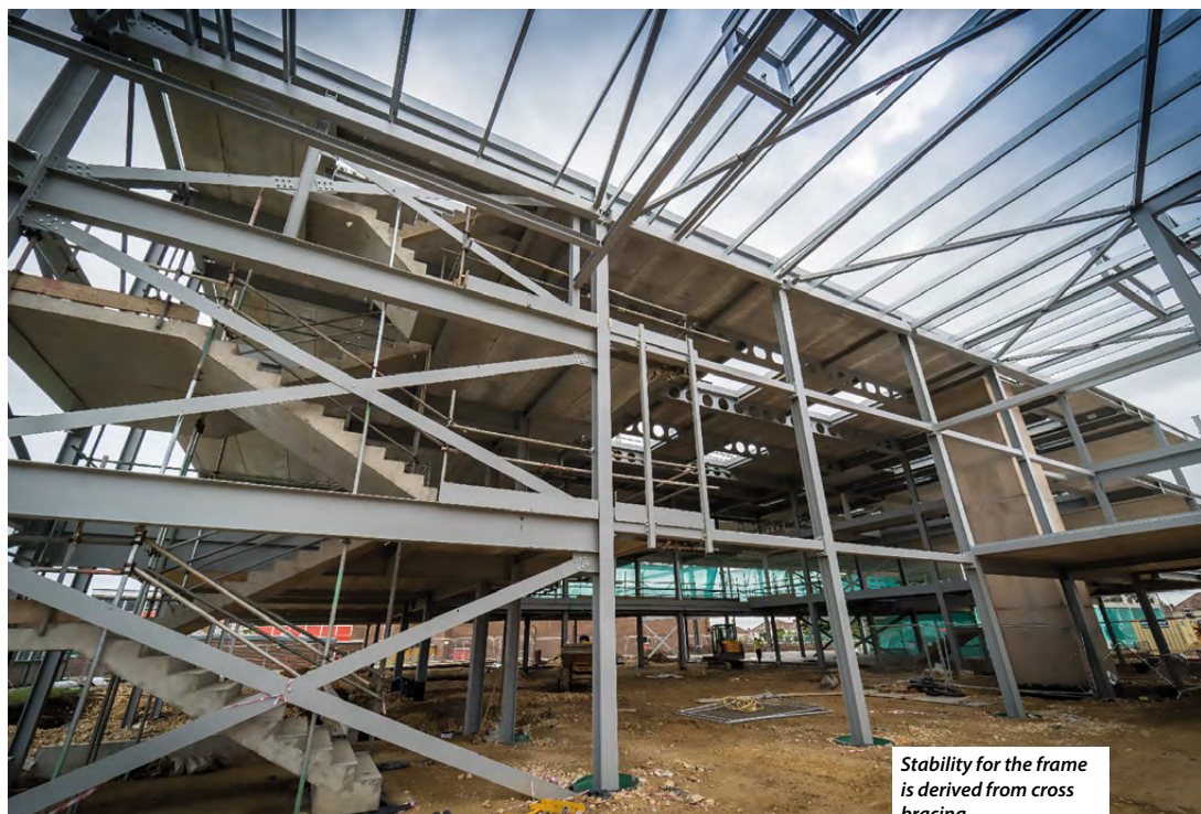
The steelwork supports precast planks to form the floors
