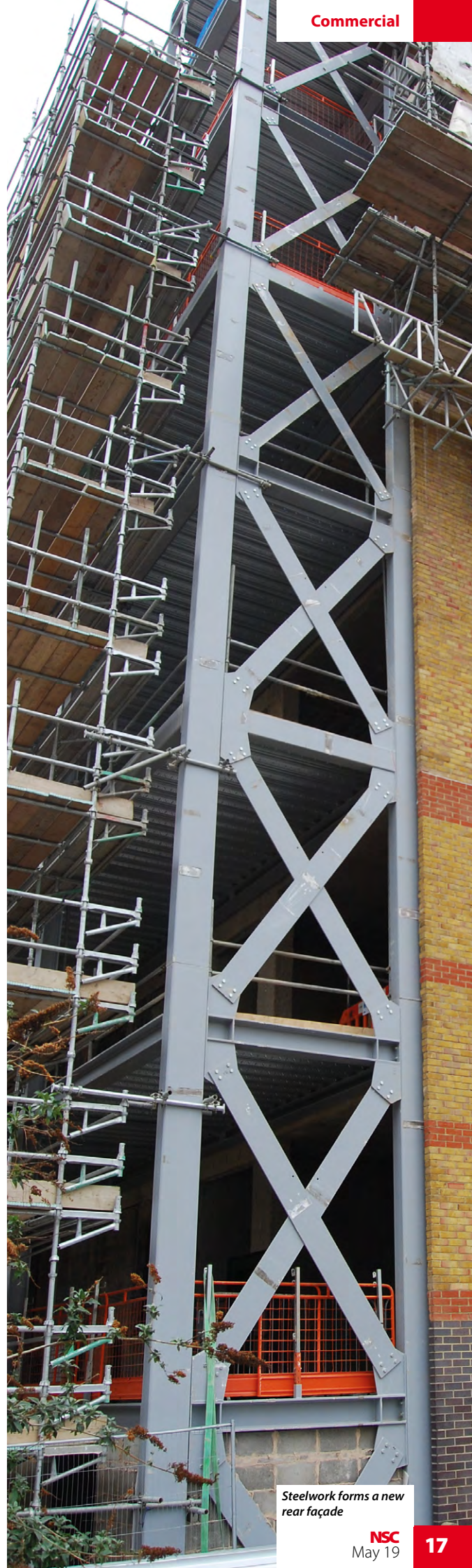
Parts of the crane bases will remain as permanent columns
