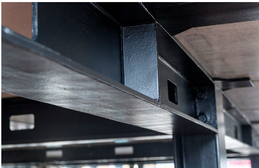
Once the steel was erected it was all repainted to get a high-quality decorative finish to suit the exposed design
