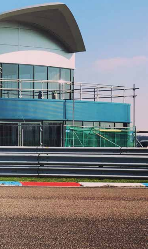
The hospitality suite is part of a larger redevelopment at Thruxton
