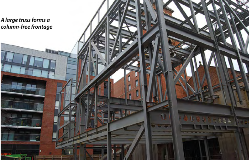
The steel frame connects to the existing church building
