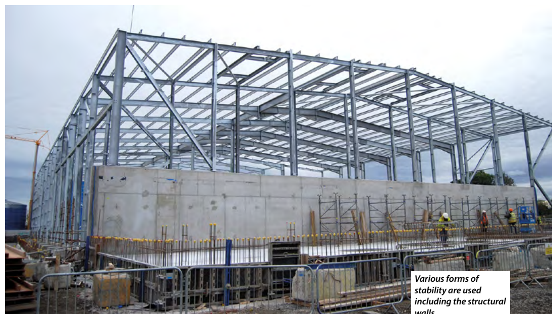
The structure is a propped portal frame
