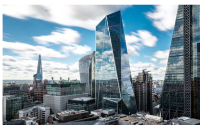
Steel was the only viable choice to form the distinctive scalpel design at 52 Lime Street
