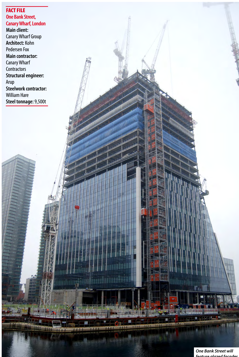
Steel erection progresses on the structure's upper floors
