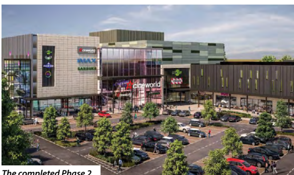
The completed Phase 2
