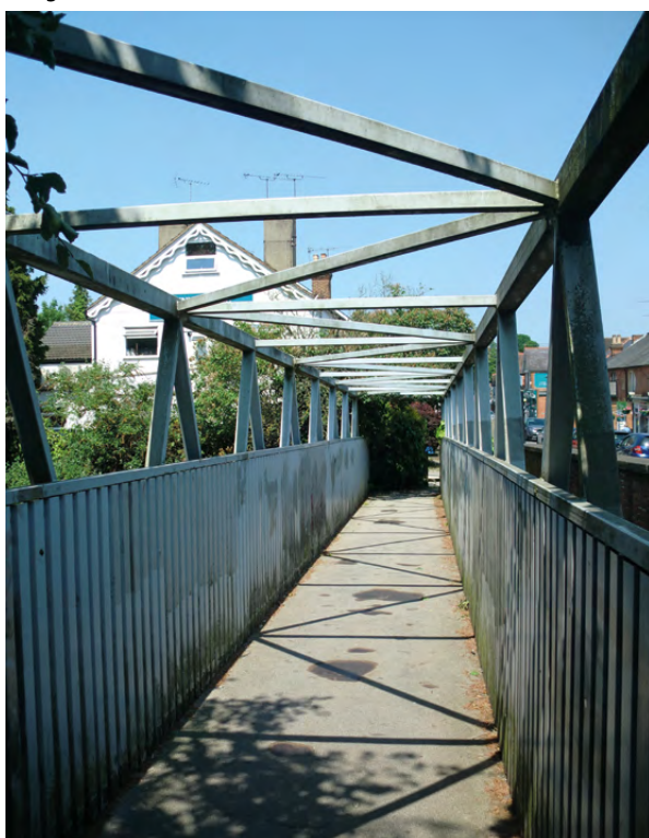
Figure 1: Truss bridge with bracing between the compression chords
