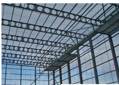
Cellular beams form the clear spans
