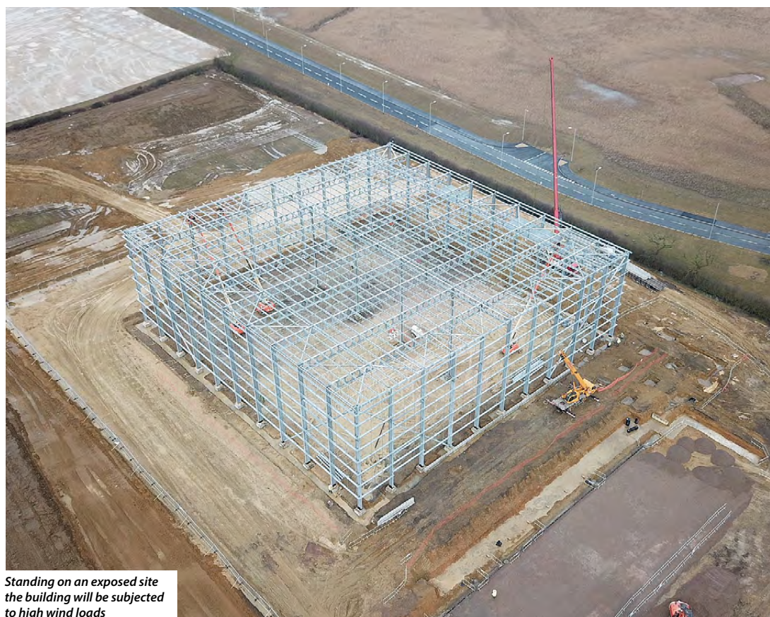
Roof bracing extends around the entire structure
