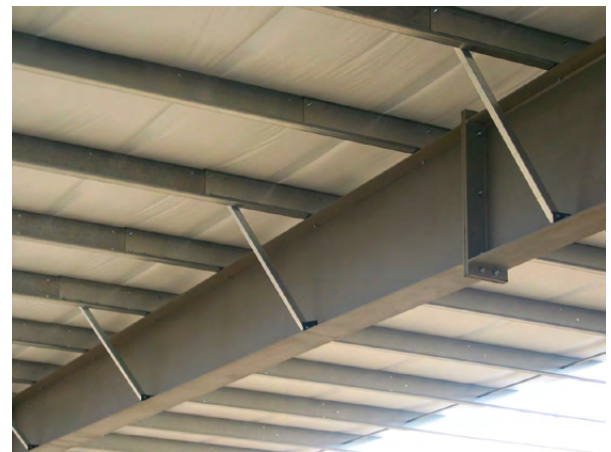
Figure 6: typical bracing to rafter
