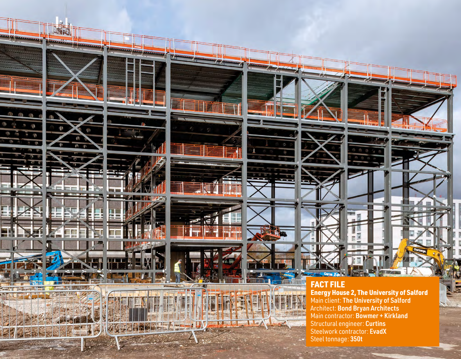
Metal decking and a concrete topping supported by cellular beams forms the structure’s uppermost level
