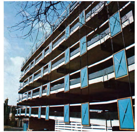
View showing beginning of ramp section of floor slab and finished panels and framing
