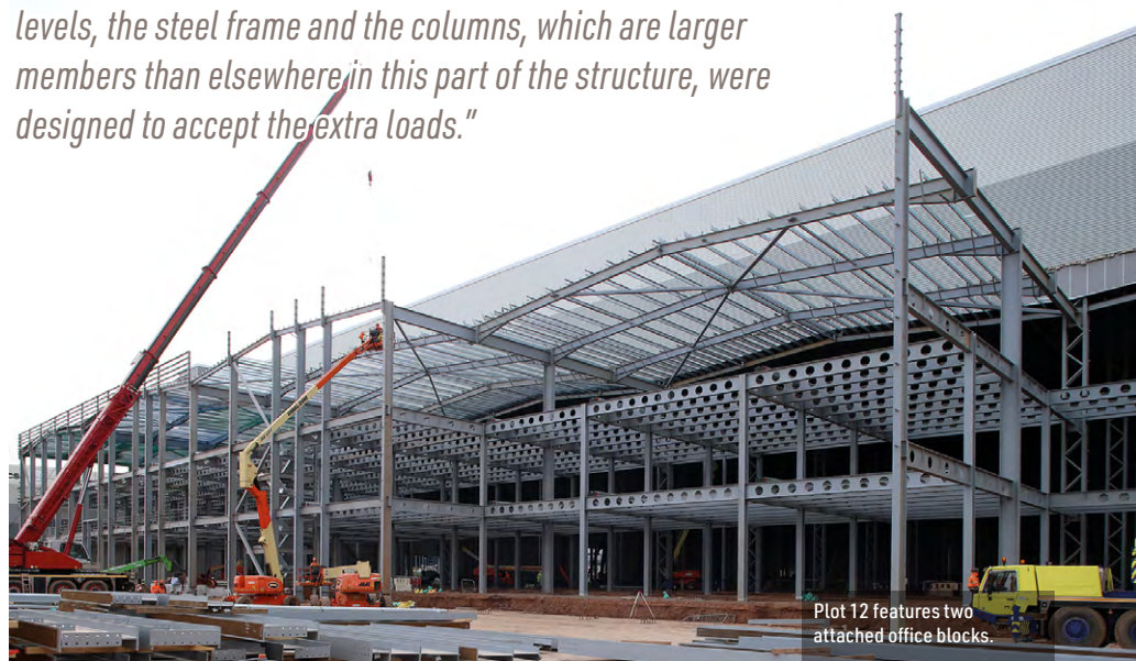
The structure's five high bay areas are 33m-high and have column-free spans of 33m.
