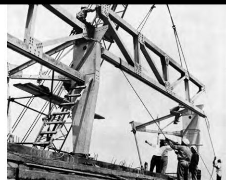
Erection of longitudinal guides between columns.
