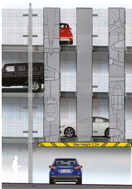
The aluminium cladding features patterned perforations depicting the town's aviation heritage.
