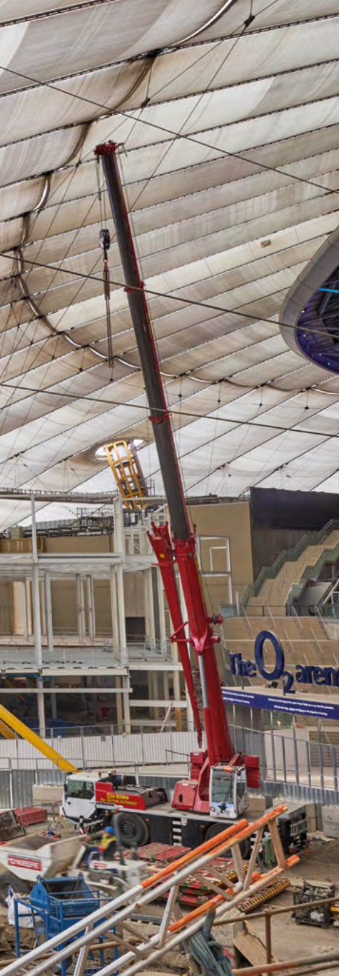
New steel connects to the existing trusses to form plant areas
