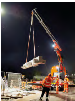
Figures 3 & 4: Countess Wear Footbridge: Left: Stainless steel cantilevers being lifted into position during a night closure Right: Stainless steel parapet posts and handrails
