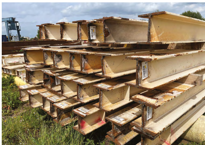
Figure 1: Recovered steel members (courtesy Cleveland Steel & Tubes Ltd)
