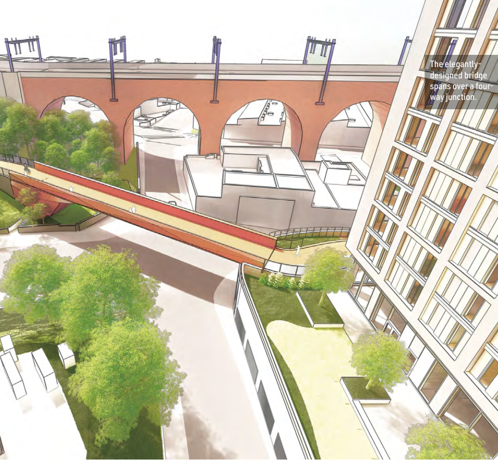
The use of weathering steel will allow the new bridge to develop a similar hue to the adjacent railway viaduct.
