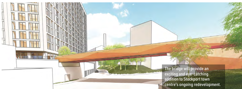
The bridge was fabricated by SH Structures in two pieces, that were welded together onsite.
