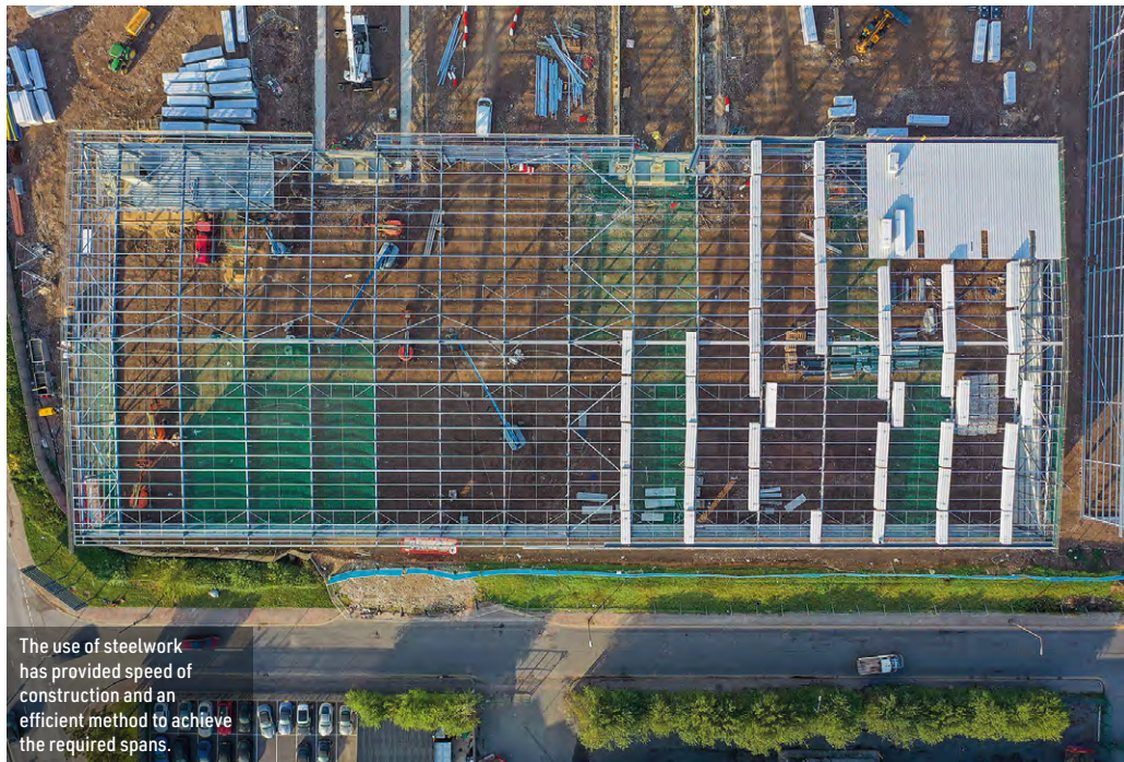
Steelwork erection nears completion on Building Two, in the foreground, while roof cladding is installed on the adjacent Building Three.
