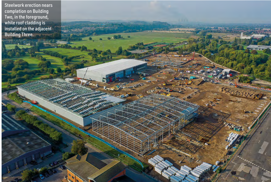
The use of steelwork has provided speed of construction and an efficient method to achieve the required spans.
