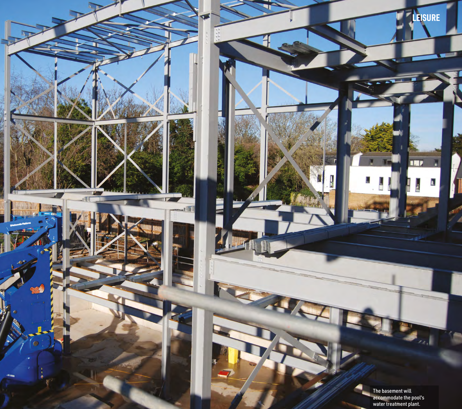
Structural steelwork was chosen as it offered the most efficient method to form the long span areas.
