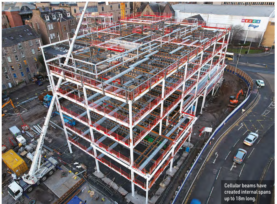
The offices have been pre-let to BT as a new regional HQ.
