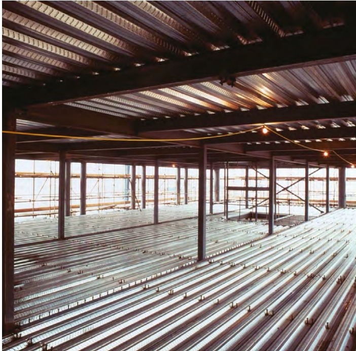
Figure 2: A continuous floor plate awaiting concrete pouring. Rows of studs indicate the beam lines, and even with continuous concrete the slabs will be designed to be simply supported at these points (at ambient temperature)
