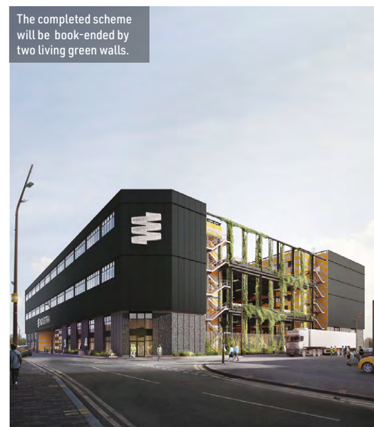
Flexibility has been designed into the project so it can be extended northwards into the adjacent plot.
