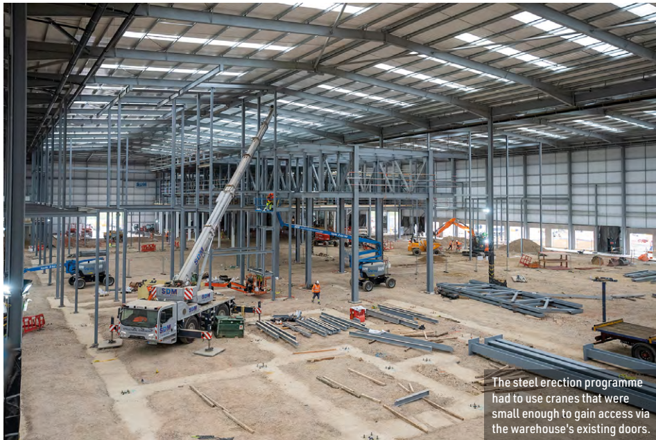
Either side of the central bridge/corridor, steelwork forms a series of manufacturing and welfare spaces.
