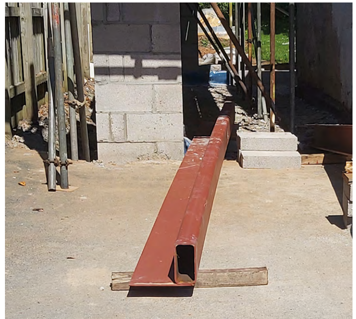
Figure 2: Torsionally stiff member for eccentric loading condition
