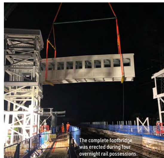
Close coordination between all stakeholders ensured the safe erection and installation of the station structures.
