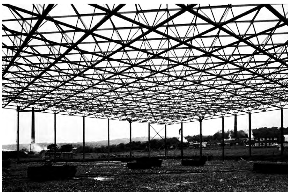
Unibat space frames for a stores building. Clear spans 50m x 50m
