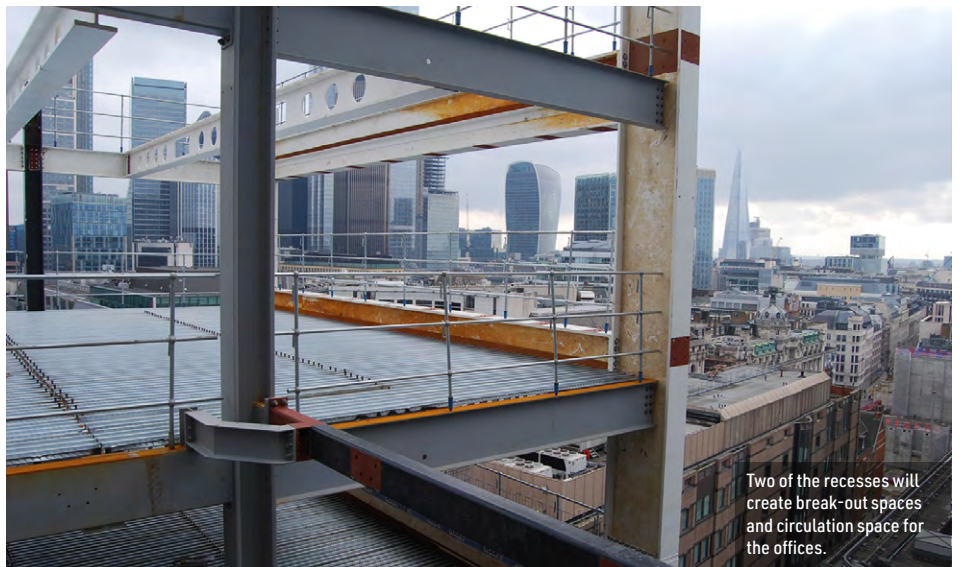
Cellular beams accommodate building services within their depth.
