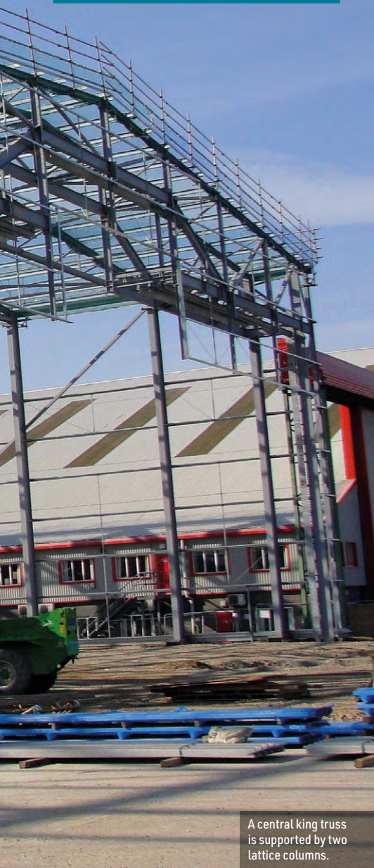
Large column-free spaces are vital for hangars and can be efficiently formed using a steel-framed solution.
