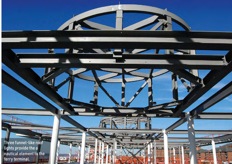
Model showing the steel frame for one of the roof lights.
